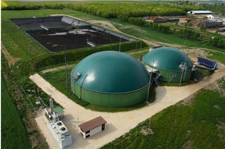
The investment reached the 70% preparedness. The two towers (which contain the reactors of the plant) are 21m high and each has 4.000 cubic meter capacity. Primarily they will use the biogas to generate electricity, this will provide the electricity for the Tettye Forrásház (which deals with water and wastewater utilities). Furthermore if the town can buy buses with biogas fuelled, the biogas plant will be able to provide their fuel.
